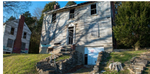
Lock House at Dam # 1
